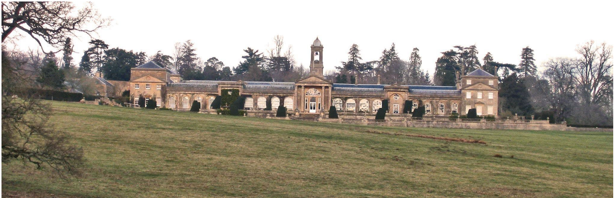
Bowood House as it stands
