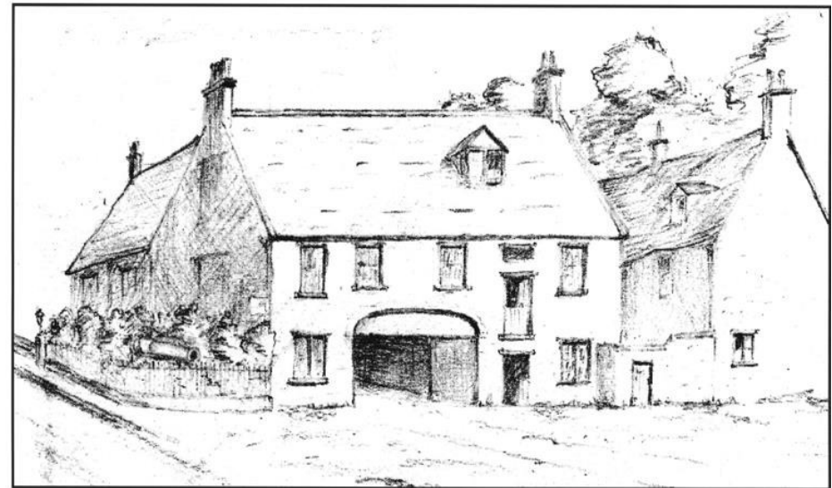
A drawing of the Calne Town Mill which once stood on the site of the Town Hall
