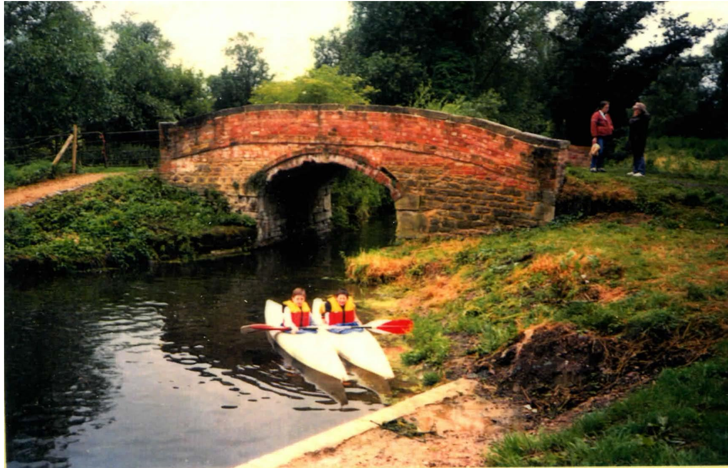
CALNE - Chaveywell Bridge restored.
